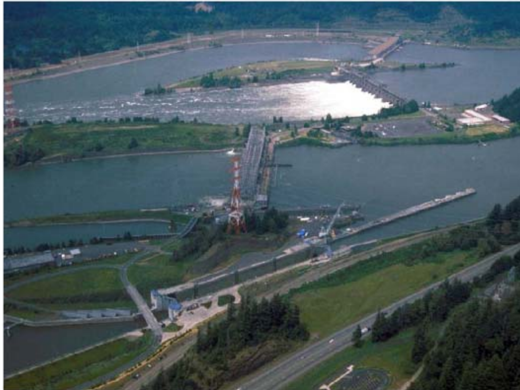
Figure 2-1 Bonneville Lock and Dam
